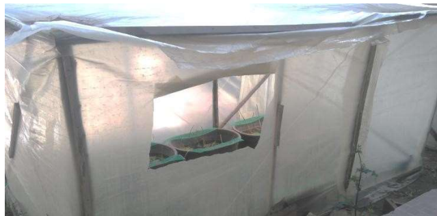
Figure 1. Floating Macrophyte Filter Greenhouse Source: Diana Quintana, 2017
